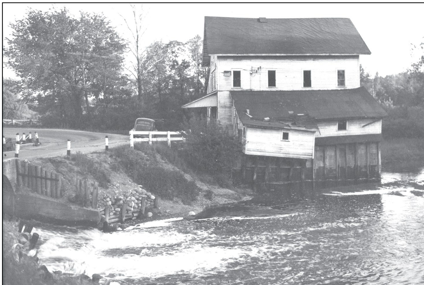
Above: Colby Mill, photographer unknown, taken circa 1940s, LaGrange Township. Donated to the Cass County (now Cass District) Library by Charles Springsteen, July 1978.
